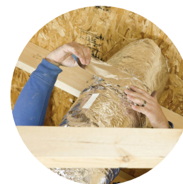
Sealing leaky air ducts
