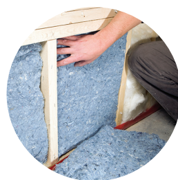
Adding insulation and sealing air leaks
